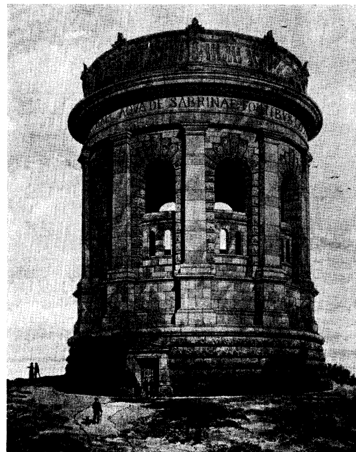
Norton, UK. Courtesy: Liverpool Water Supply Unit, Liverpool Corp., City Engineers Dept., Bootle, Merseyside. Norton Tower is a massive masonry structure of Roman Doric design, built of local sandstone. The inscription, large enough to read from ground level, translates: "This water, derived from the sources of the Severn, is brought to the City of Liverpool, a distance of 80 miles, through the mountains and plains of Wales and the intervening country, at the cost of the municipality, in the year of our Lord 1892".
